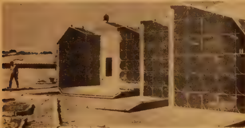
Old 55 gallon oil barrels filled with water, painted black, absorb heat from sun during day. In the evening side panels (seen laying on ground) are drawn shut. Barrels give off warmth all night long heating most of house.
